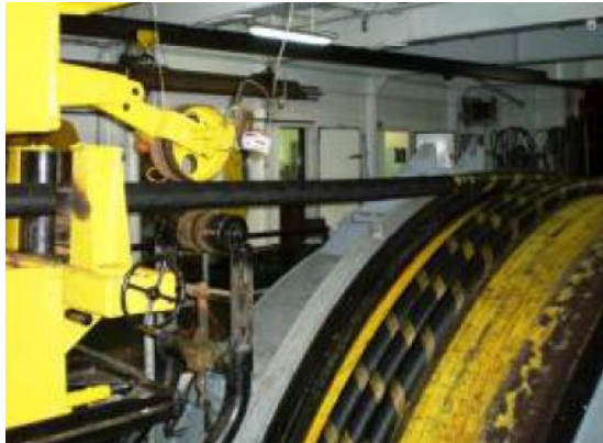
Sea trial test of laying facilities
