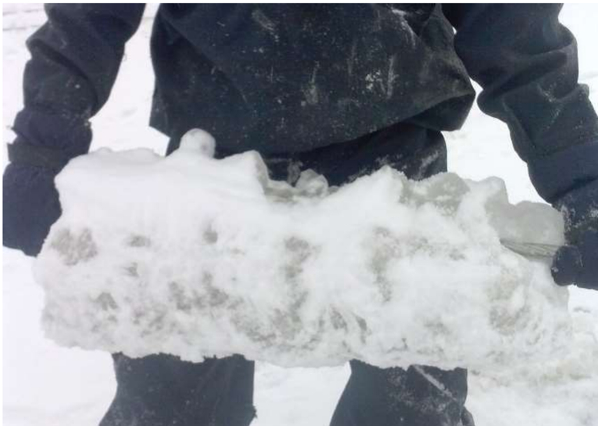
Figure 1: An icy shell on a DV 110 kV phase-conductor of Cerkno –Idrija transmission line
