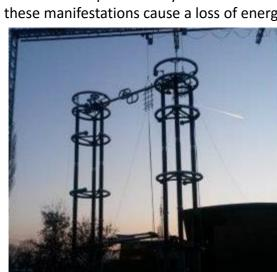
Fig. 3 Knee type disconnector1000-1200kV
