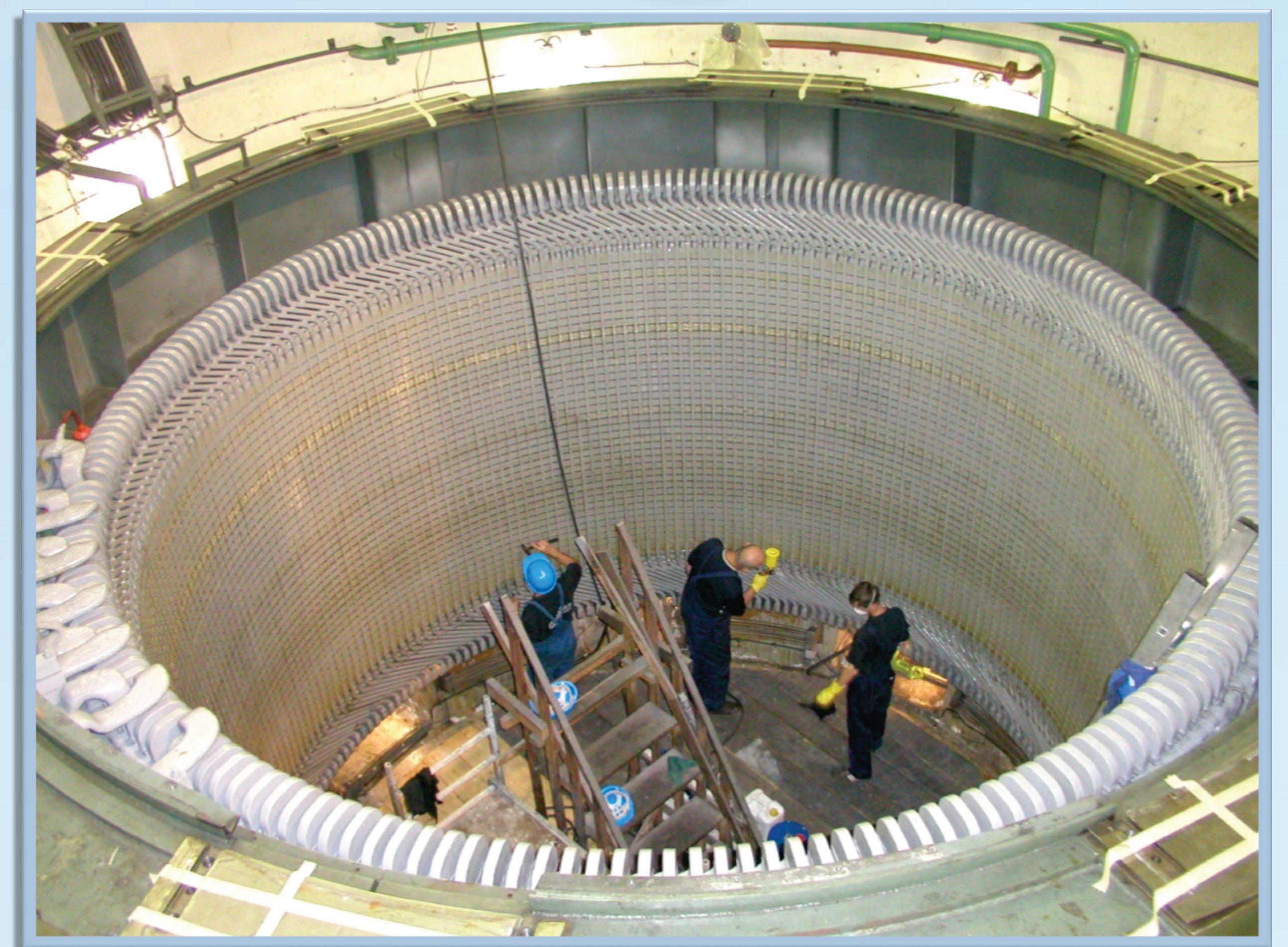
HPP Zakučac, Works on generator stator Upgrade 2 x 120 MVA & 2 x 150 MVA to 4 x 160 MVA
