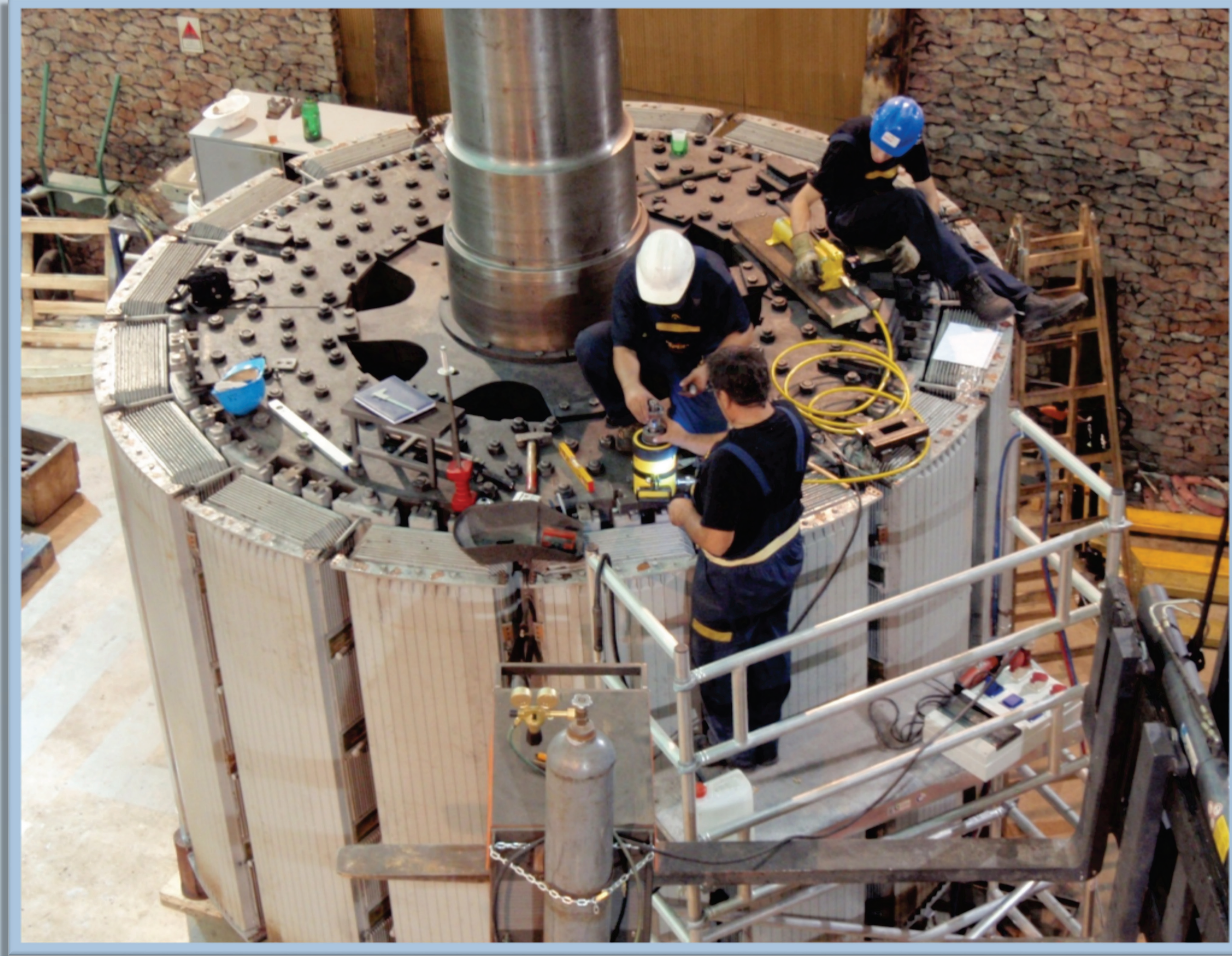
HPP Rama, Refurbishment of generator rotor Upgrade from 90 to 100 MVA
